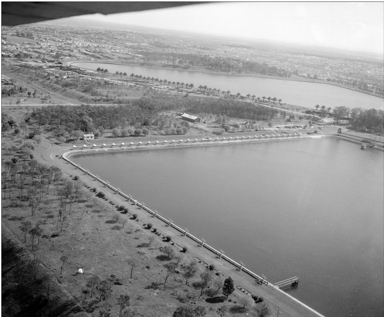
Figure 12: View looking southwest across the two Potts Hill water reservoirs in 1953, showing Christiansen's solar grating arrays along the banks of the eastern reservoir. The E-W array consisted of thirty-two elements and the nearer N-S array just sixteen elements (RAIA 3475-1).
