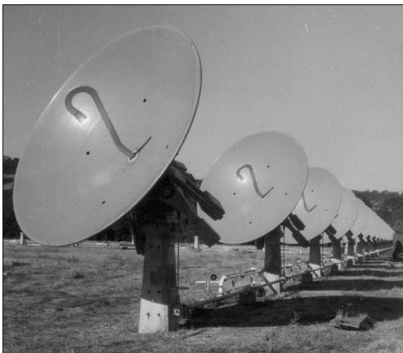
Figure 37: A close-up showing the design of the metal dishes, feeds and mountings (courtesy: TIFR Archives).
