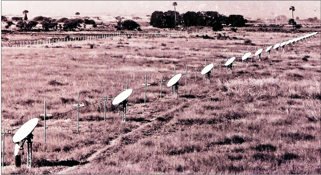
Figure 43: View of part of the east-west grating array, consisting of twenty-four 1.8-m diameter dishes and built at Kalyan, near Mumbai, in 1965 (courtesy: TIFR Archives).
