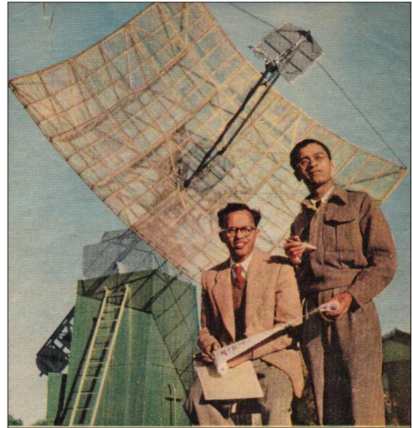
Figure 20: Govind Swarup (left) and R. Parthasarathy (right) at Potts Hill field station in 1954. At the time, this 16 × 18 ft ex-radar antenna was being used to map the distribution of neutral hydrogen in our Galaxy (after Illustrated Weekly Times of India , 1954).
