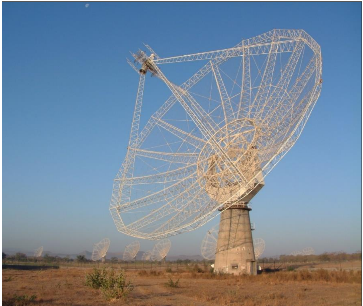
Figure 52: A close up of one of the 45-m antennas, with six others in the background (courtesy: TIFR Archives).
