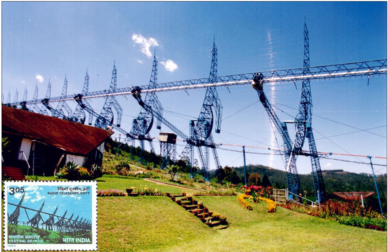
Figure 47: Another view of the Ooty Radio Telescope; reflections of sunlight by 1,100 stainless steel wires are seen on the right. The inset bottom left shows an Indian stamp featuring the ORT (courtesy: TIFR Archives).
