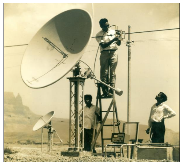
Figure 44: A close-up of two of the Kalyan array antennas, with R.T. Kapahi adjusting the transmission line (courtesy: TIFR Archives).
